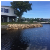
Rip Rap Seawall
