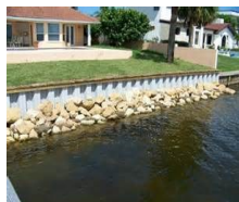
Vinyl Seawall with Rip Rap
