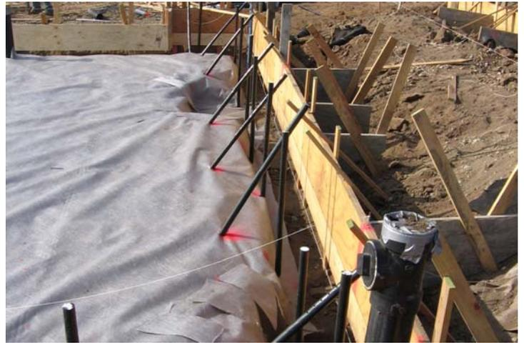
2. Have the vapor retarder contractor spray directly to the **VaporStake™**. Since the **VaporStake™** is made of PVC and is round like a pipe, the vapor retarder contractor can use the same details that are used to seal around the plumber's pipe penetrations.
