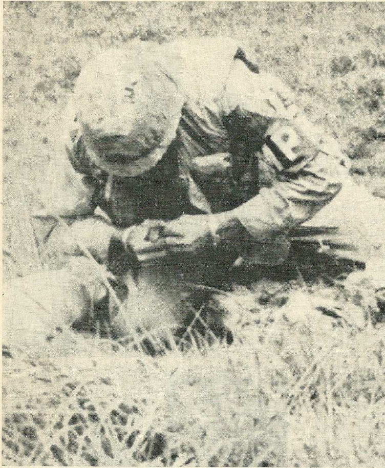
After discovering a Viet Cong tunnel at the top of Mang Yang Pass, Spc. 4 Donald Peyton of B Company prudently uses a fragmentation grenade to check for occupants.
