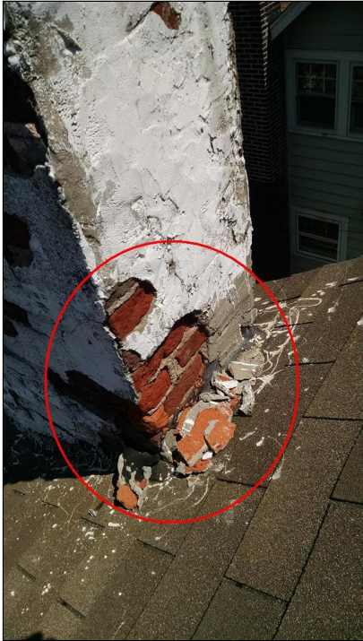
6.5 Item 3(Picture) Bricks spalling
