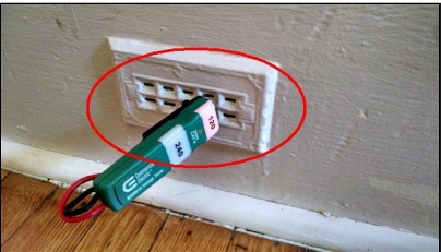
8.7 Item 5(Picture) Live outlet in living room wall
