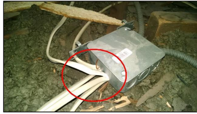
8.7 Item 9(Picture) Wires entering the box
