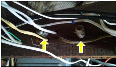
8.7 Item 3(Picture) Knob and tube wiring porcelain insulators
