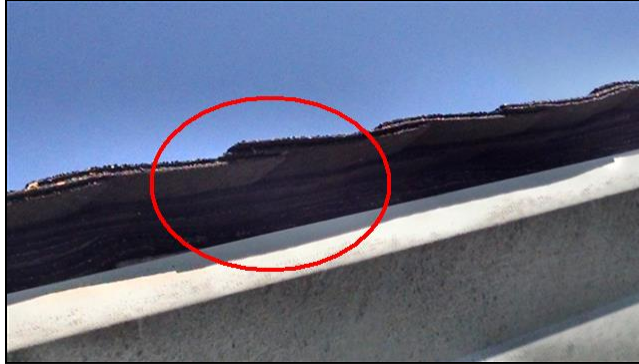
6.0 Item 3(Picture) 3-4 layers of shingles
