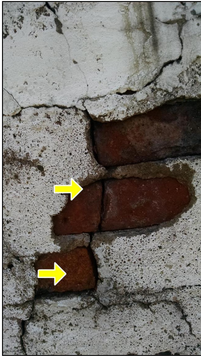
6.5 Item 5(Picture) Bricks cracked
