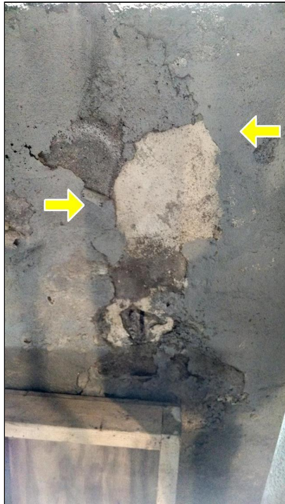
5.2 Item 1(Picture) Paint/parging flaking off
