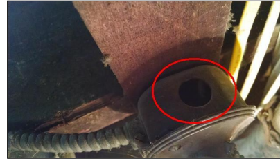
8.7 Item 2(Picture) Light fixture missing knockout
