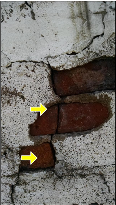
6.5 Item 5(Picture) Bricks cracked
