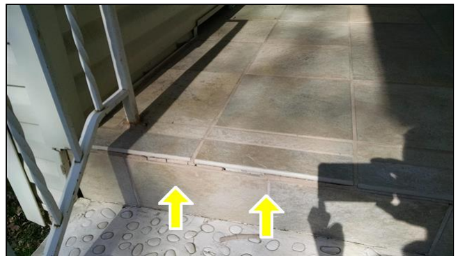
2.9 Item 2(Picture) Grout joints cracked and tiles loose
