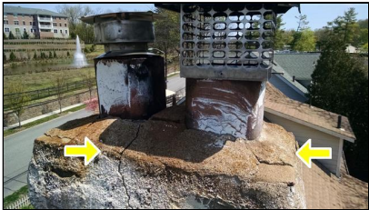
6.5 Item 4(Picture) Crown cracked
