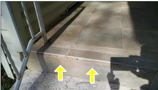
2.9 Item 2(Picture) Grout joints cracked and tiles loose
