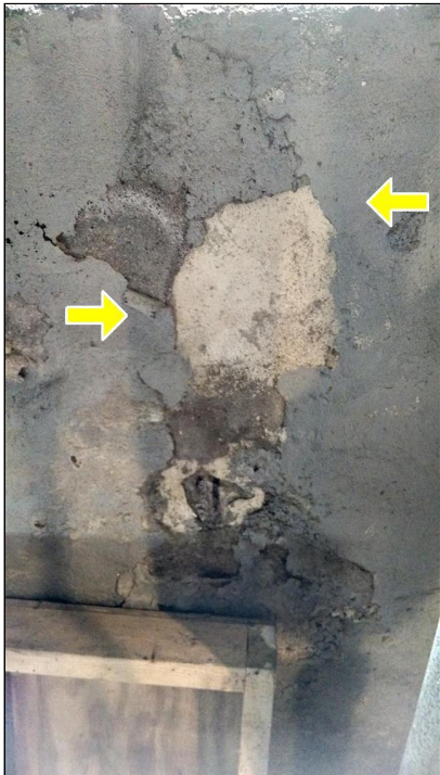
5.2 Item 1(Picture) Paint/parging flaking off
