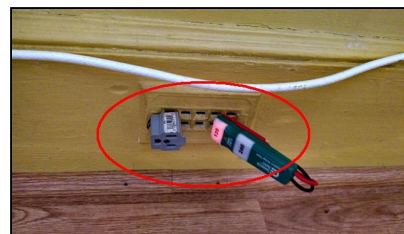
8.7 Item 7(Picture) Live outlet in front bedroom wall
