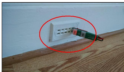
8.7 Item 6(Picture) Live outlet in middle bedroom wall
