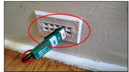
8.7 Item 5(Picture) Live outlet in living room wall
