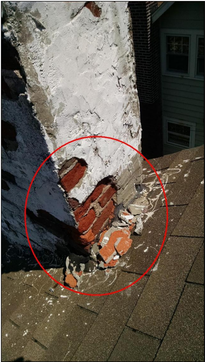
6.5 Item 3(Picture) Bricks spalling
