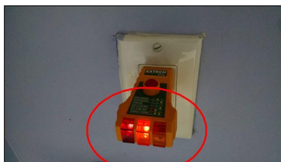
8.8 Item 7(Picture) Bathroom GFCI outlet
