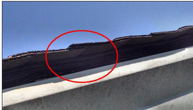
6.0 Item 3(Picture) 3-4 layers of shingles
