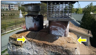
6.5 Item 4(Picture) Crown cracked
