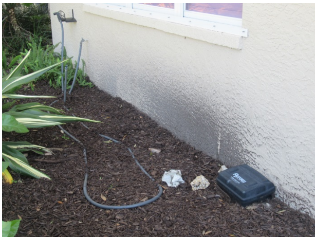
Stucco coated walls – damage to the paint finishes evident
