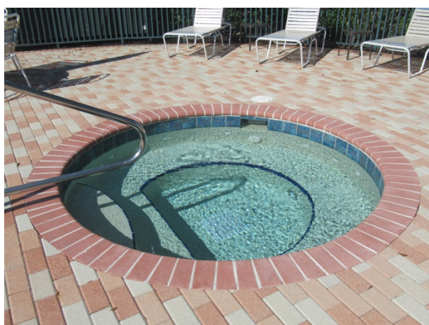
Pool finishes – deterioration of the plaster evident
