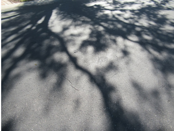
Asphalt pavement streets – deterioration of the seal coat application and cracks evident
