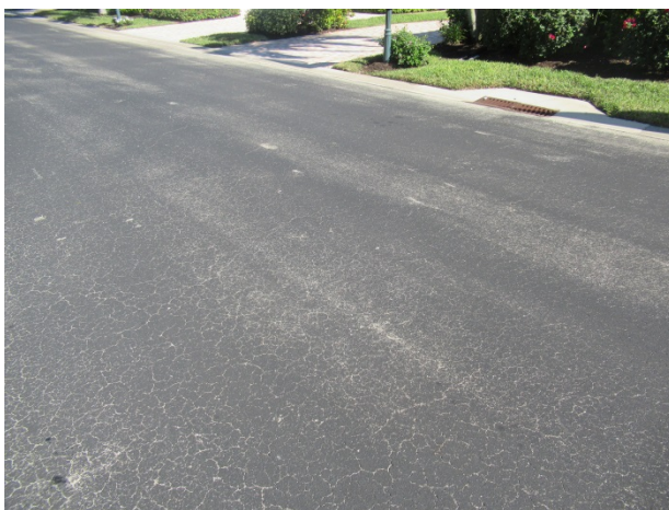
Asphalt pavement streets – deterioration of the seal coat application and cracks evident
