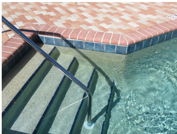
Pool finishes – deterioration of the plaster evident
