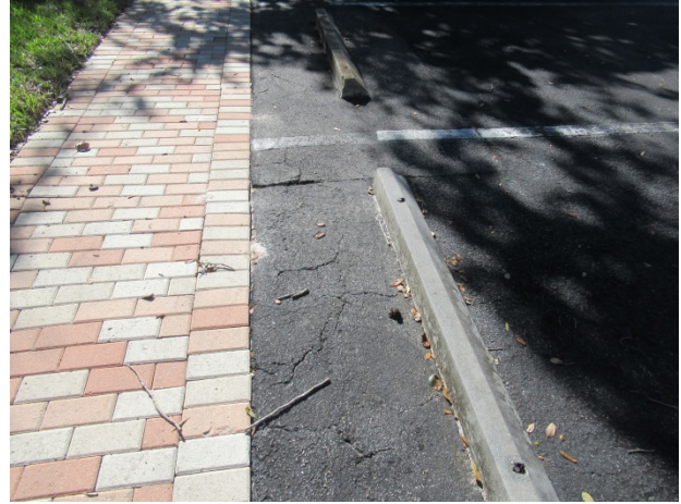
Asphalt pavement streets – cracks evident
