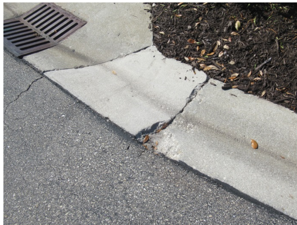
Concrete curbs and gutters – damage to the concrete evident
