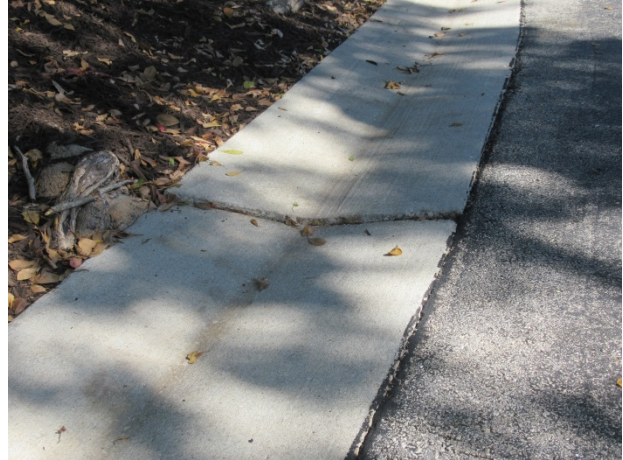
Concrete curbs and gutters - uplift evident
