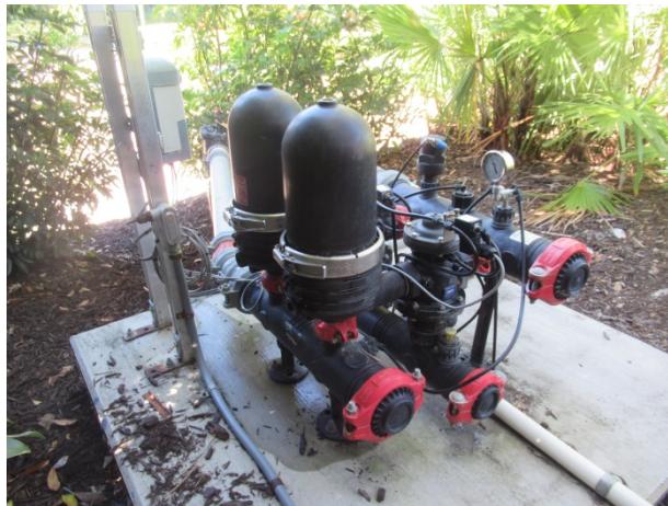
Automatic filtration system
