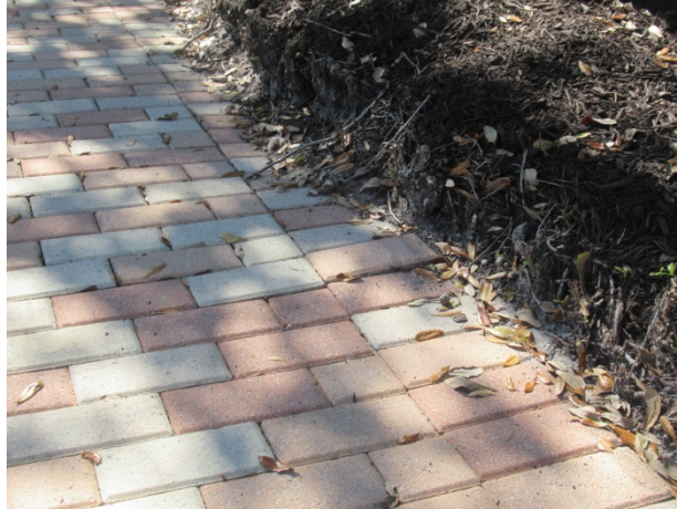
Masonry pavers – uplift evident
