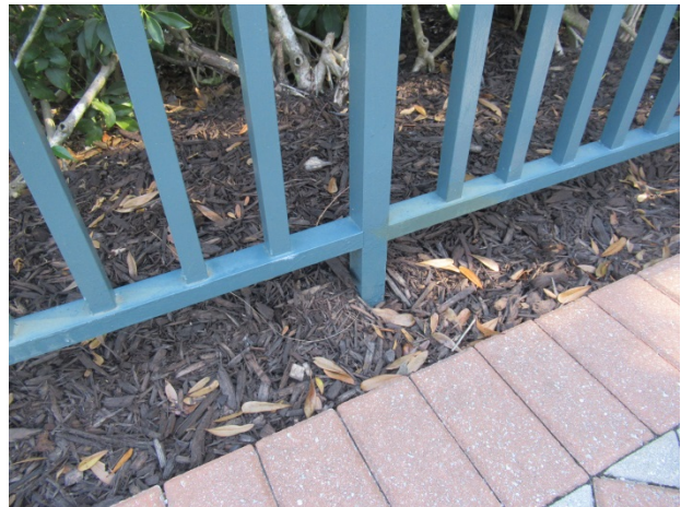
Aluminum fence – deterioration of the paint finishes evident
