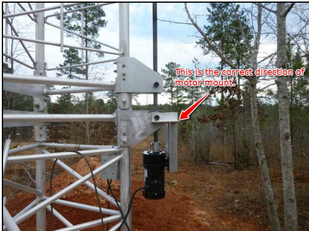
Pictured Above: Correct position of motor mount, side view. Mount is not symmetrical from left to right; therefore mount must be in a reverse 'F' position, not in a forward 'F' position, when looking at it from the side
