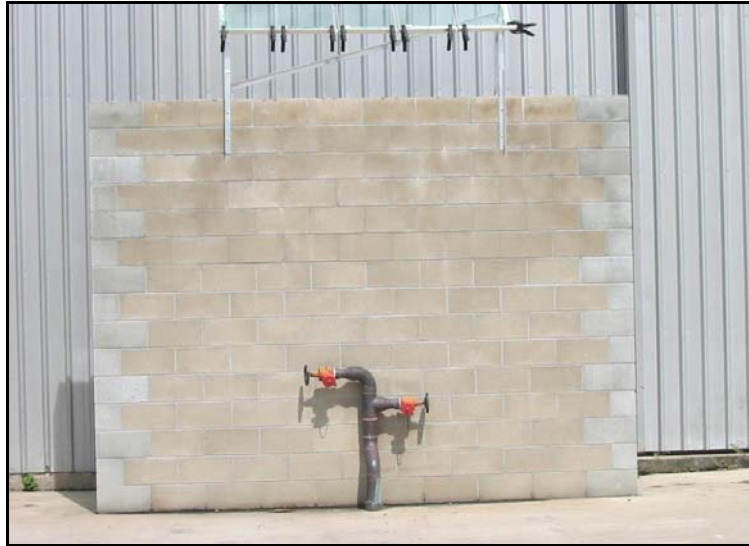
Figure 3 – Protection of External Hydrant
