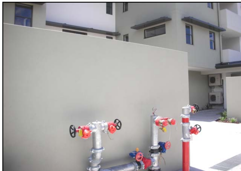
Figure 4 – External Booster Protection
