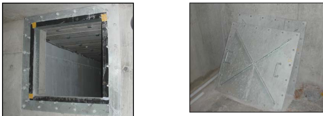
Figure 9 – Bolted Access Hatch
