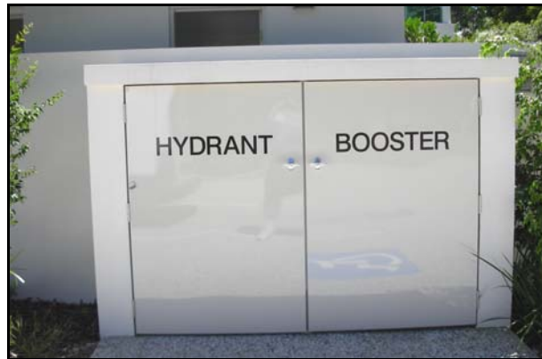
Figure 5– Stainless Steel Booster Cabinet
