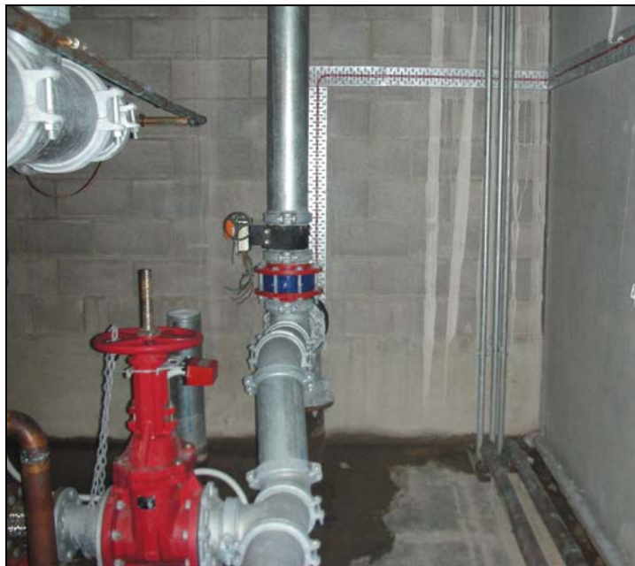
Figure 12 – Pump Room Leakage
