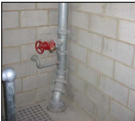
Figure 1 – Hydrant in Fire Isolated Stair
