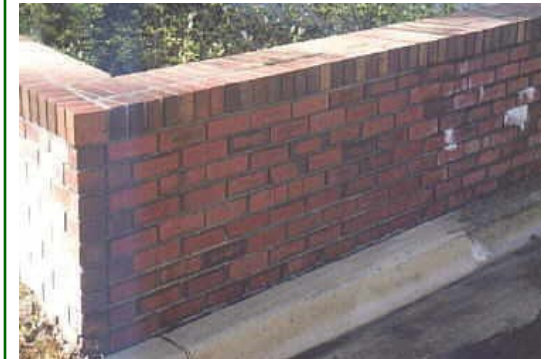
Before & After Efflorescence Removal
