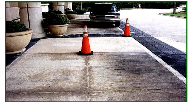
Before & After Oil and Grease Removal
