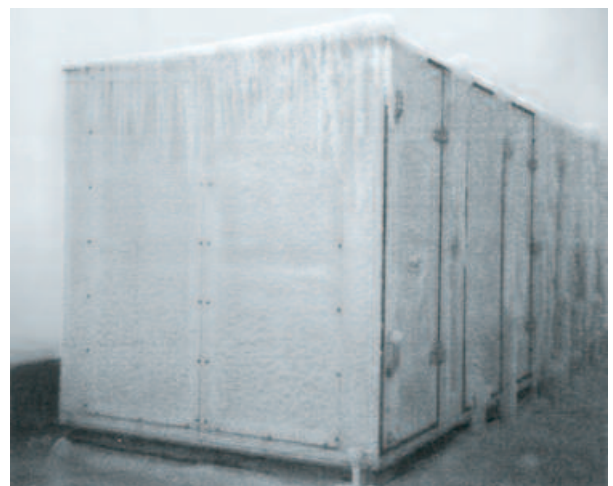
Conditions do not always have to be 'extreme' for extreme problems to arise. These images of totally ice-bound air intakes were taken in northern Germany in ambient conditions of around 0 °C.
