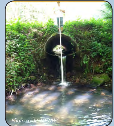
Perched culvert (pre-project)
