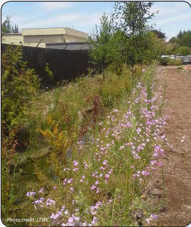
Stormwater filtration swale at Gibson Steel
