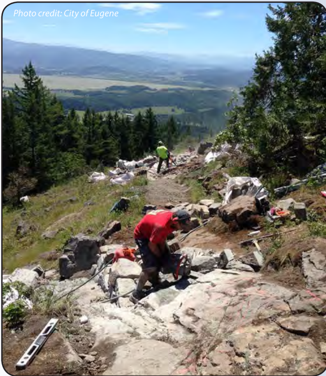
Trail construction on Spencer Butte
