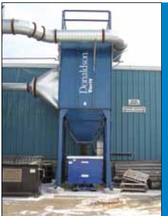
54MBTH8 at a cabinet shop on wood dust, from cutting, moulding and sanding
