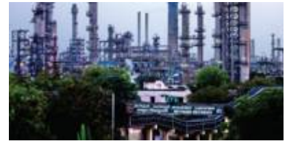
Mathura Refinery 8.0 MMTPA
