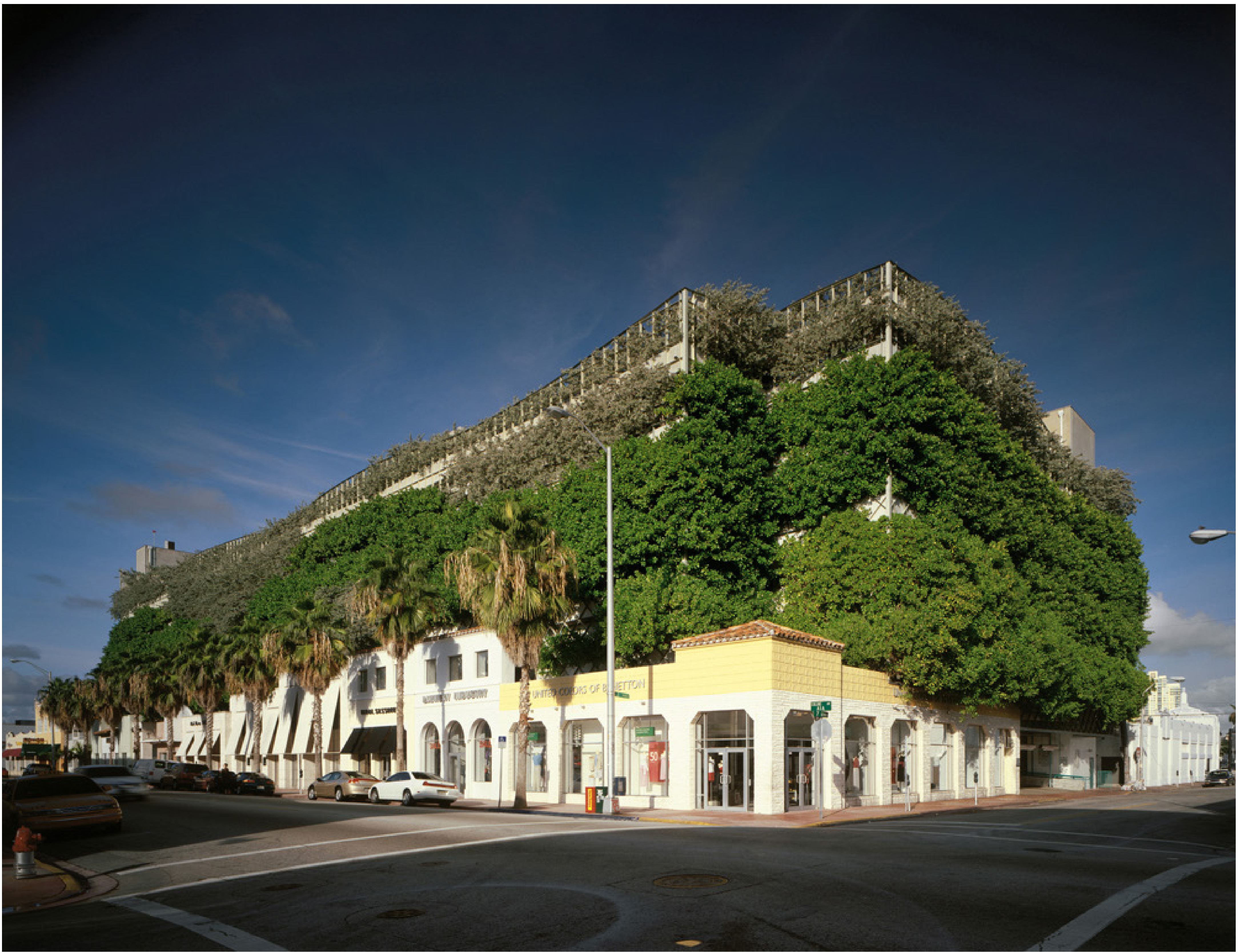
Commercial Ground Floor Parking Garage with Vegetated Wall Miami, FL
