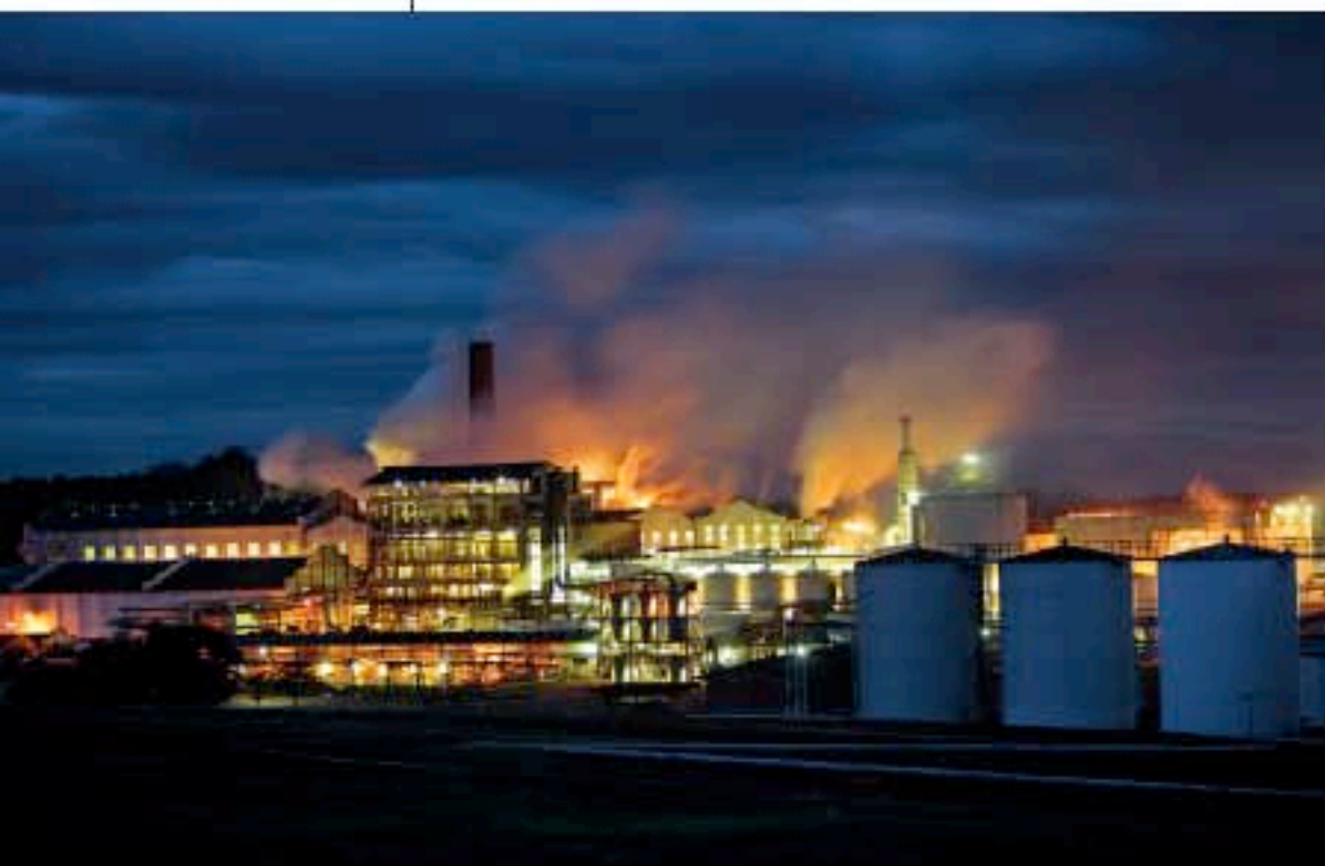
Lighting up the night near Pradópolis, Brazil, Usina São Martinho is one of the largest ethanol refineries in the world, producing 300 million liters annually—without relying on fossil fuel or electricity from the grid. For heat and power, the plant burns sugarcane waste.
