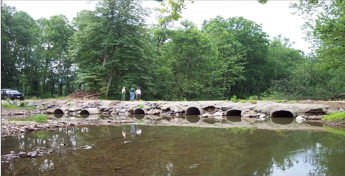
Photo 49. Water body is an RPW. This photo shows water flowing through a culvert. Culvert does not affect the jurisdictional status of the water body.
