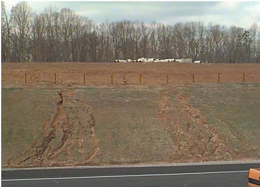
Photo 60. These erosional features are small channels eroded into the soil surface by runoff.
