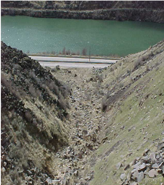
Photo 24. Unnamed ephemeral tributary, Boise County, ID. Flow is piped under Highway 21 (and into the Boise River).
