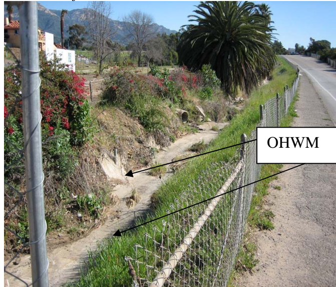
Photo 51. A roadside ditch excavated wholly in uplands, CA. Feature is not jurisdictional under CWA.
