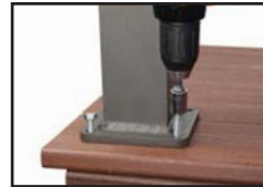
Fasten Post to Deck Surface
