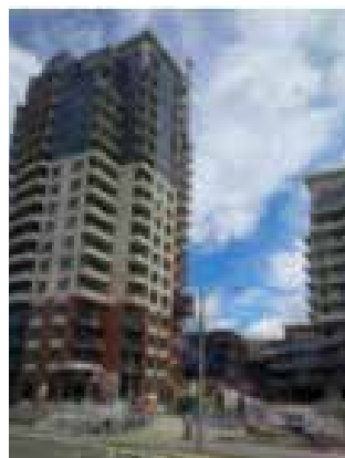
50 Fontenay court under construction at Scarlett Road and Eglinton, 17 floors
