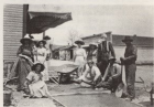
Building the cement sidewalk from the depot to the center of town with donated labor.
