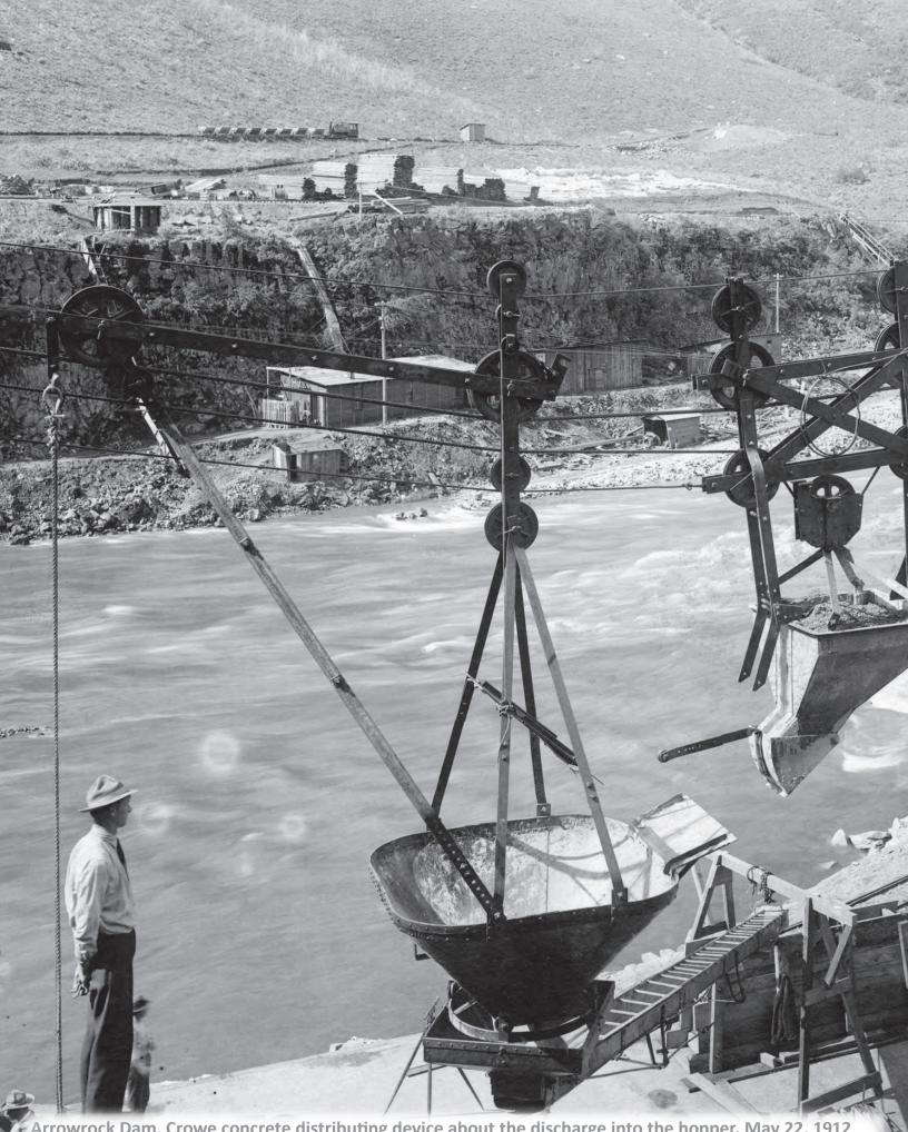
Arrowrock Dam, Crowe concrete distributing device about the discharge into the hopper. May 22, 1912 Photo Credit: Idaho Historical Society, 61-164.88
