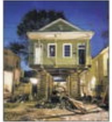
STAFF FILE PHOTO BY DAVID GRUNFELD A double house on Cherokee Street in the Tulane/Loyola university area was raised to make room for more apartments in January 2020. The raised is house is now near completion.
