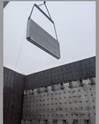
Baffles Replaced Through Open Stack
