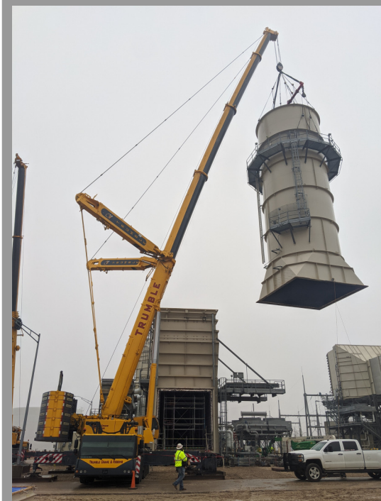
Turn-Key Stack Removal
