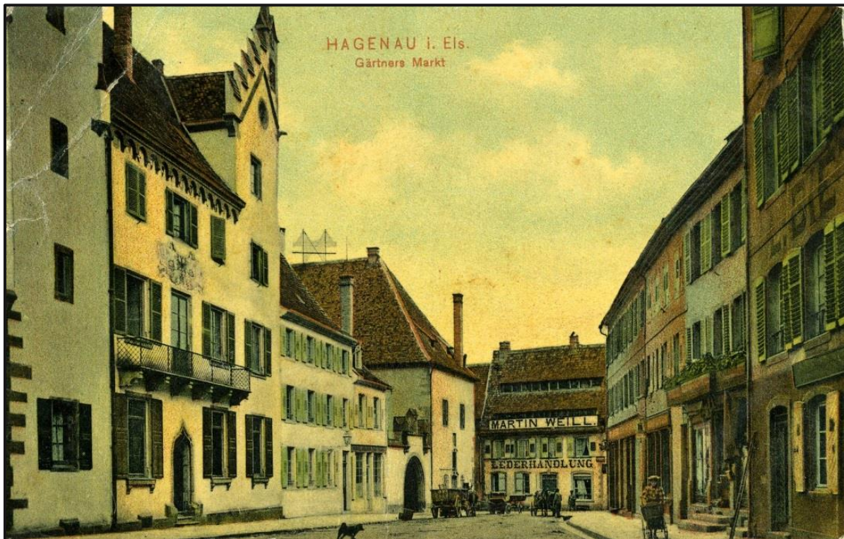
Chancellery Building, Hagenau, Built 1484
