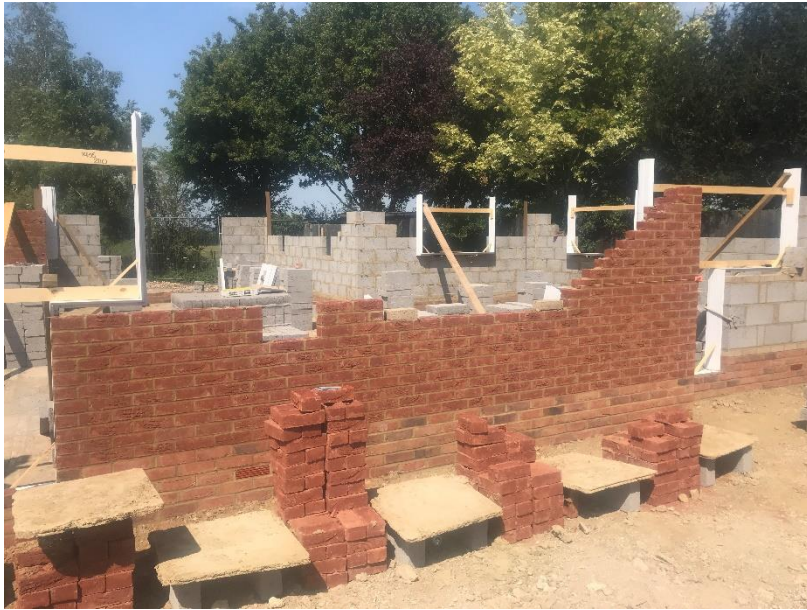
Face brickwork Plot 4
