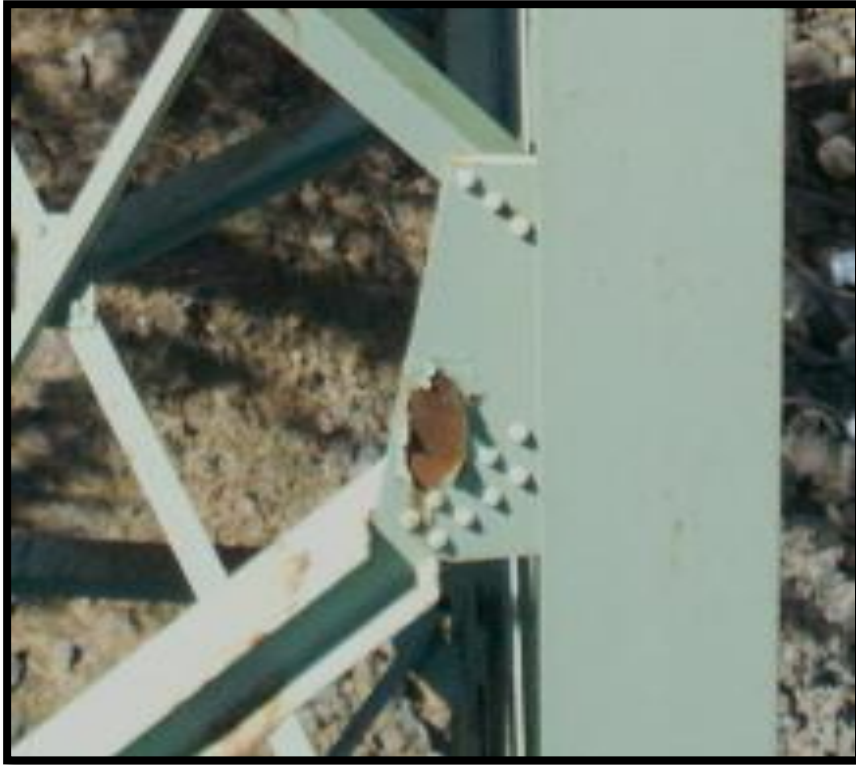
Paint Failure
