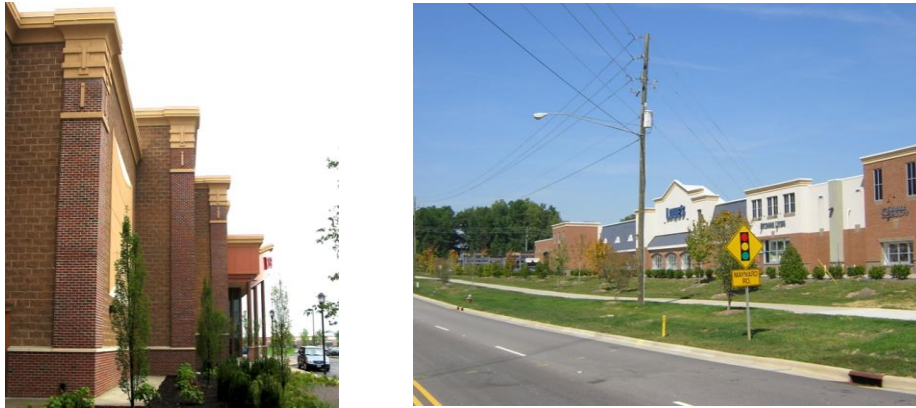
Figure 26.01 The buildings in the above images contain pilasters, cornices, and a series of facade setbacks (recesses) to visually break up the appearance of large facades.
