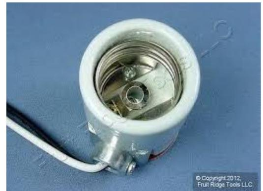
This is the part I love telling people. Go to the light and stick a plastic spoon into the light socket. Using the spoon, catch the metal tab and bend it down slightly. What you have done is put the tab back into a position to make contact with the light bulb. Don't forget to turn the breakers back on. If the problem persist, call Robart Electrical Services.
