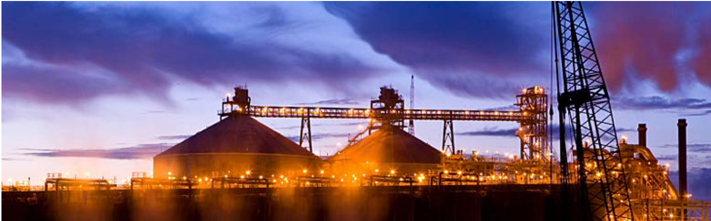
YARWUN 2 REFINERY STAGE 2 - AUSTRALIA
