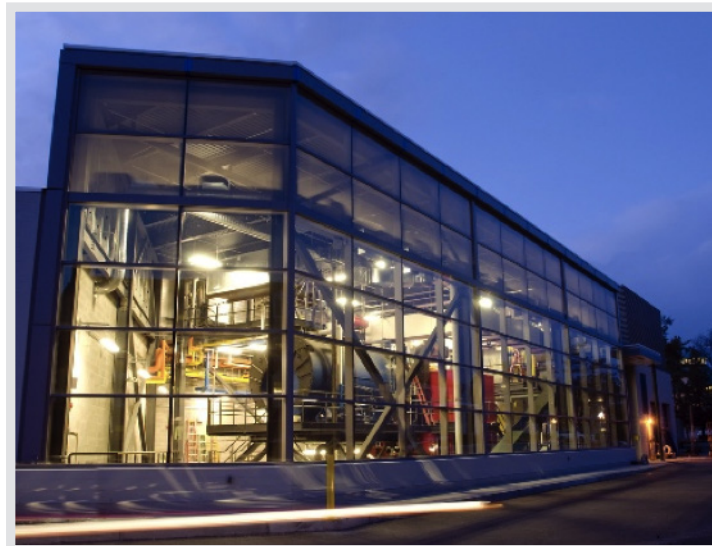
Middlebury College's $12 million biomass gasification plant moves the college closer to carbon neutrality.
