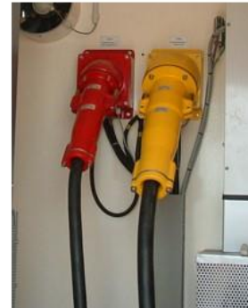
Power Cables 1 kV x 160, 240 or 320 Amp
