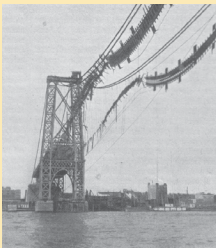
Damaged by fire while under construction in 1902
