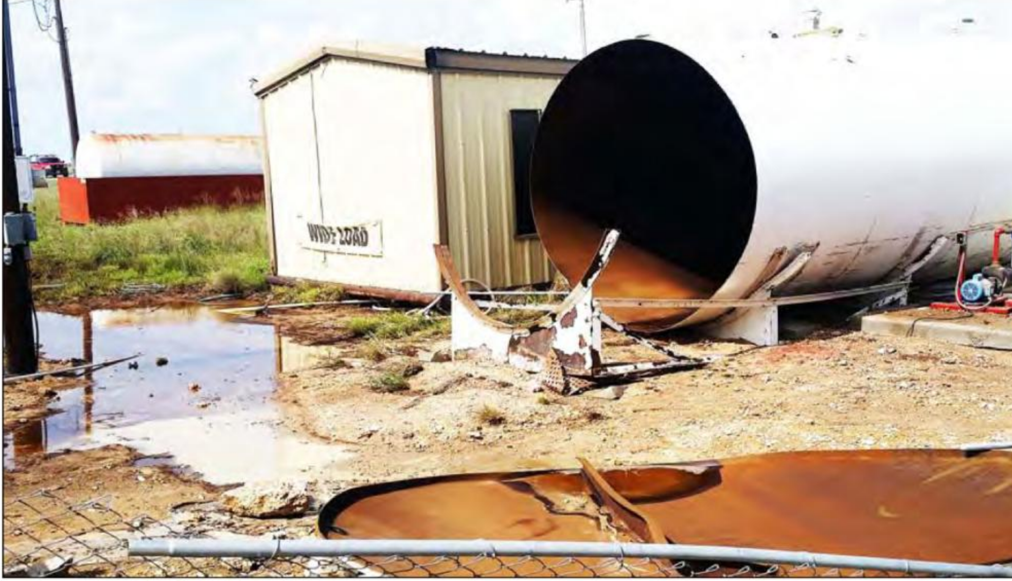
CATASTROPHE AVOIDED – A 10,000-gallon fuel tank at the Colorado City Airport was being filled when a malfunctioning vent caused the back end of the tank to blow off. Approximately 9,000 gallons of jet fuel ended up on the ground, but no injuries were sustained in the accident. Photo courtesy of Rick Goodney.
