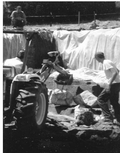
Mechanical removal of boulders at Locality I.
