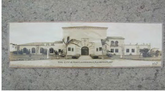
The original plant
