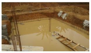
Mid-March brought us to the point where we could begin pouring the slab. While final surface preparations were being applied to the cistern walls, we began laying out the rebar that would support the slab.
