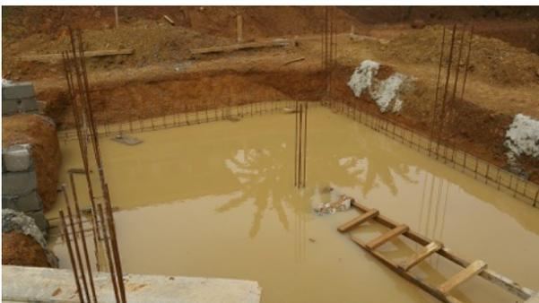
Mid-March brought us to the point where we could begin pouring the slab. While final surface preparations were being applied to the cistern walls, we began laying out the rebar that would support the slab.
