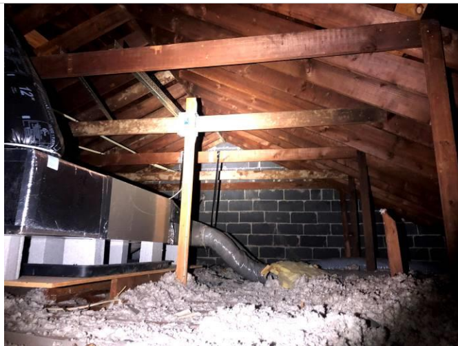
3. Roof rafters in attic of Gable-framed building
