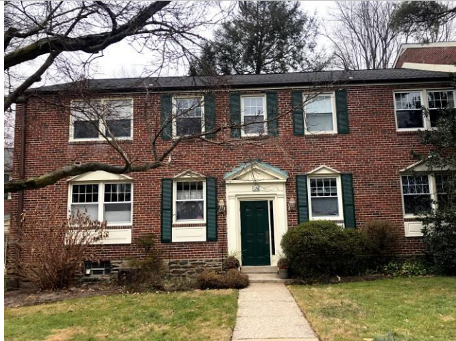
1. Front view of typical gable roof building.
