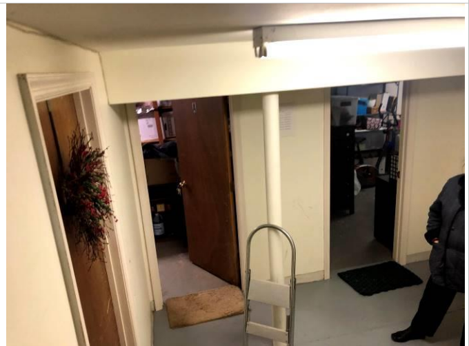
4. Steel column in basement supports load bearing wall above.
