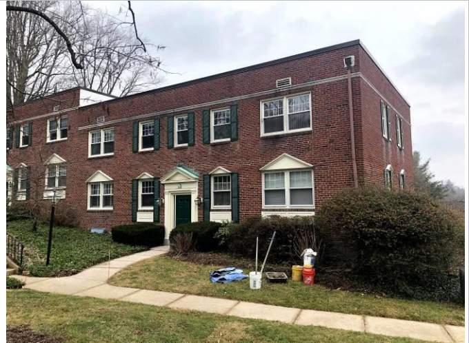
2. Front view of typical flat roof building.
