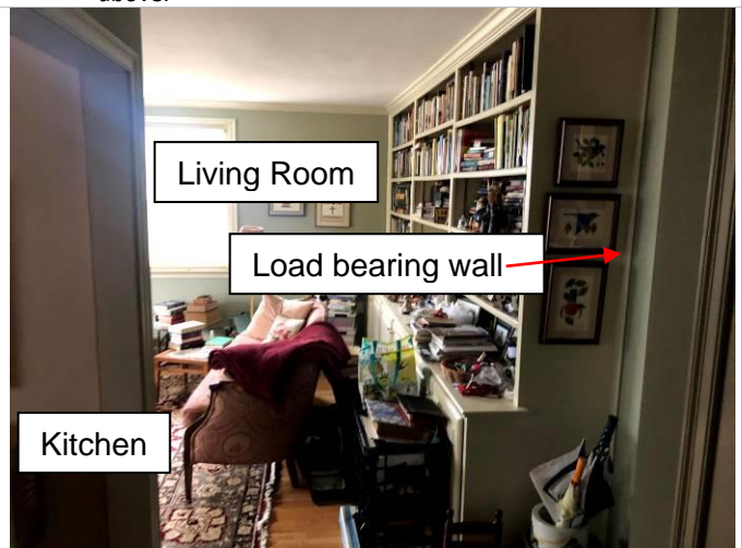
6. View inside two-bedroom unit showing load-bearing wall and wall separating kitchen and living room.
