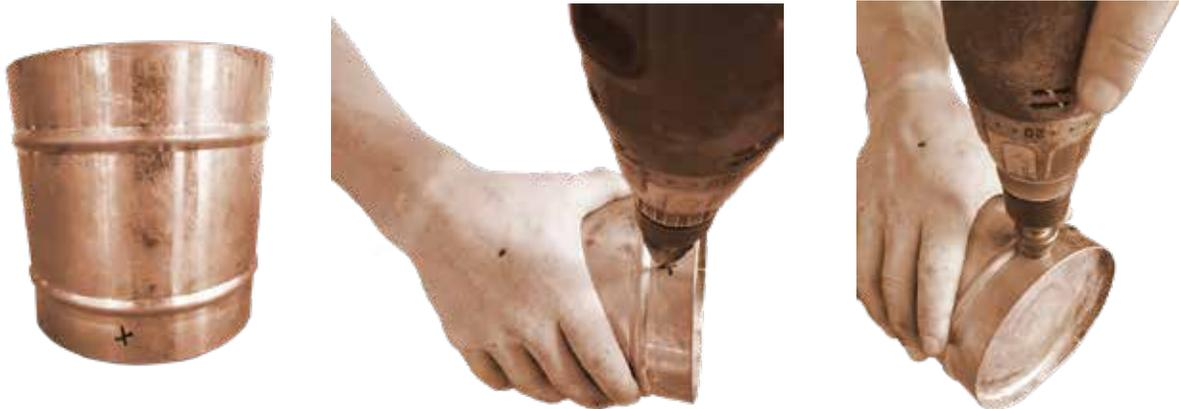
**When you heat up these pieces, it is different that heating the copper up and soldering! You need to heat up the piece slightly longer before applying the solder. If you apply the solder before the brass piece is hot enough to take the solder, you will end up with solder drips on the copper.**
