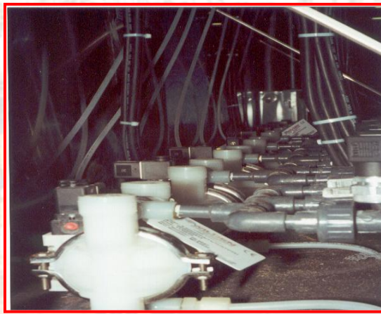
Air-actuated, multiple-injection, multiple-chemical system with AOD pumps.
