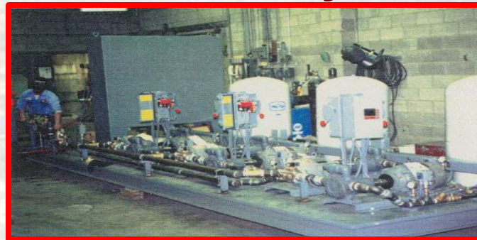
Three sets of dual gear pump systems to mix various antifreeze and water ratios, one constant speed water pump, one variable speed antifreeze pump, pressurized storage tank, control panel, mounted on a 20' x 8' steel skid.
