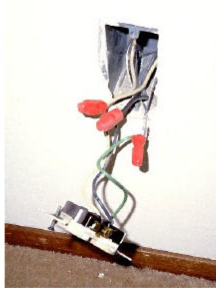
Figures 5 & 6 – Direct Wired Aluminum and Copper Pigtail with Old Style Wire Nuts
