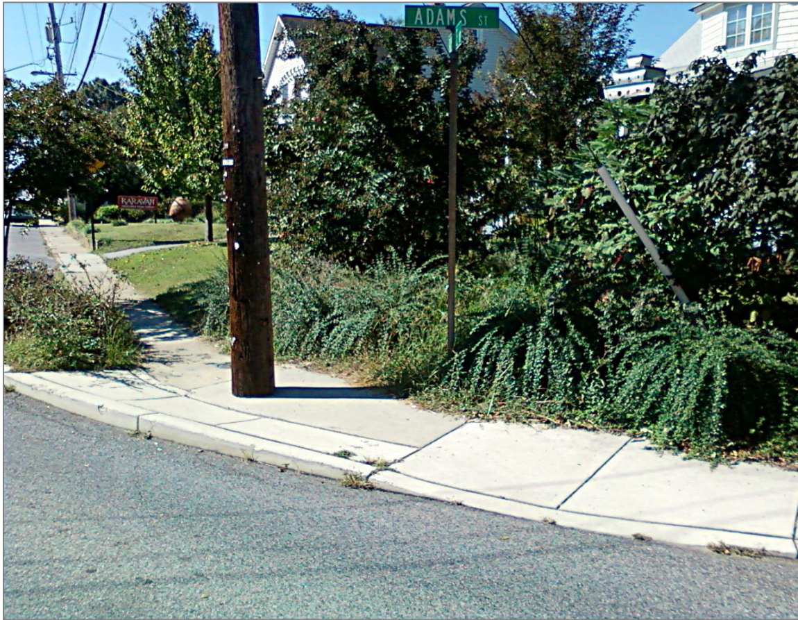
Figure 19: Pedestrian Ramp Encroachment
