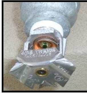
Figure 1 –Tyco Sidewall Sprinkler
