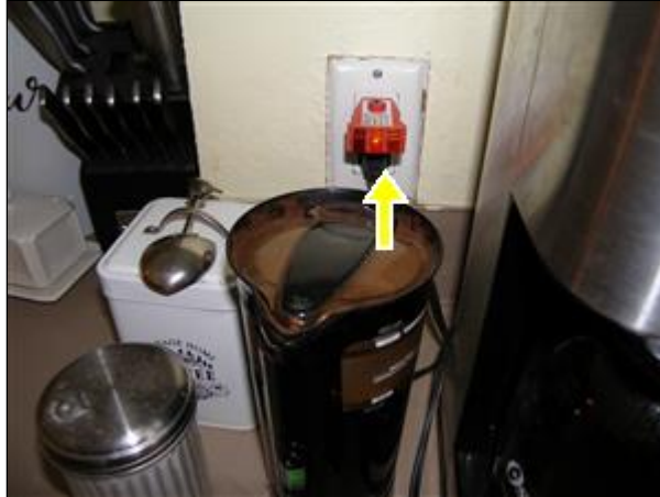
7.9 Picture 1 open ground
