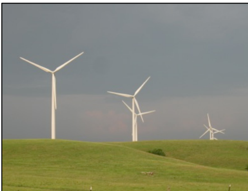
Flat Water Wind Farm in Richardson County, Nebraska.
