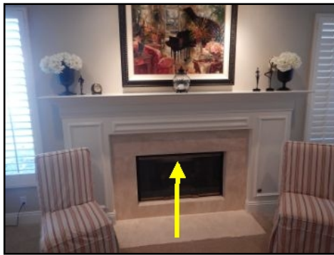
Damper Clamp missing.
