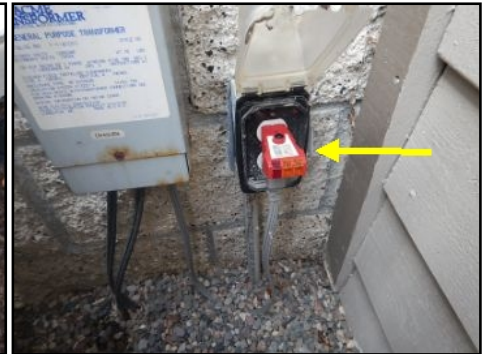
No power to receptacle behind pool equipment
