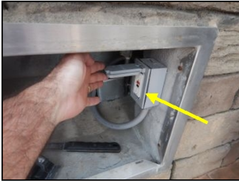
GFCI receptacle not working properly under grill
