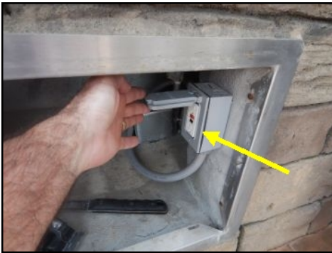
GFCI receptacle not working properly under grill
