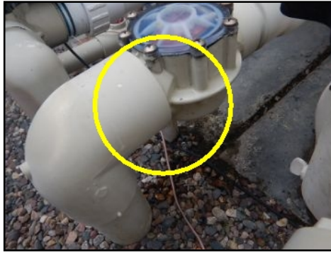
Small leak at check valve in Spa booster pipe
