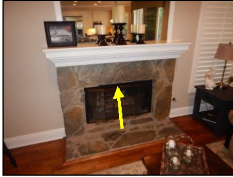
Damper Clamp missing.
