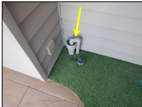
FYI - Backwash to sewer (correct piping)
