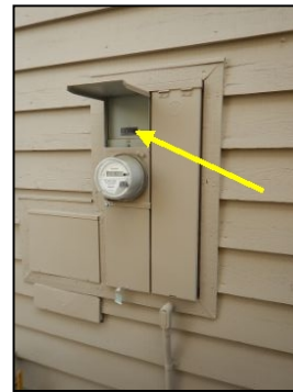
FYI - Main Electrical Disconnect Switch
