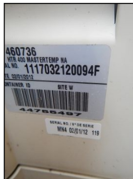
FYI - Pool Heater Data Plate
