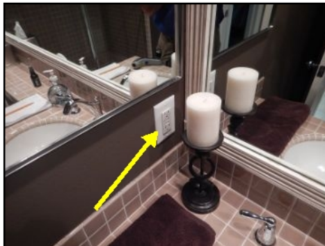
No power to all receptacles in the bathrooms
