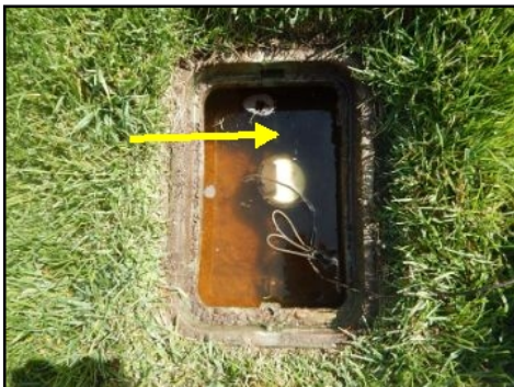
FYI - Main Water Shut-off Valve
