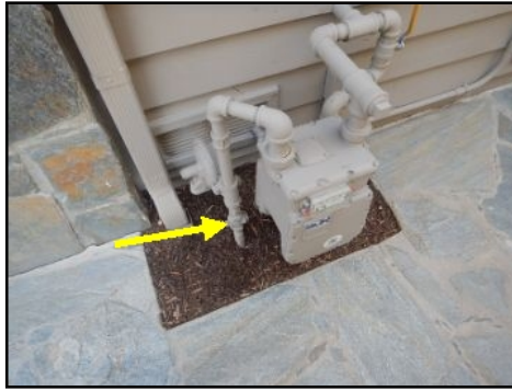
FYI - Main Gas Shut off Valve
