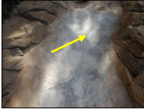
Minor shrinkage cracks on pool slide
