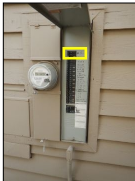
Improper 50 amp fuse for A/C
