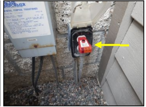
No power to receptacle behind pool equipment
