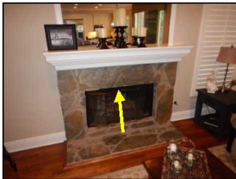
Damper Clamp missing.
