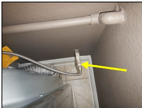
Improper gas valve in laundry room
