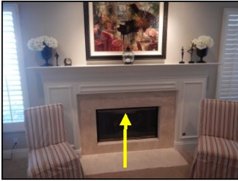
Damper Clamp missing.
