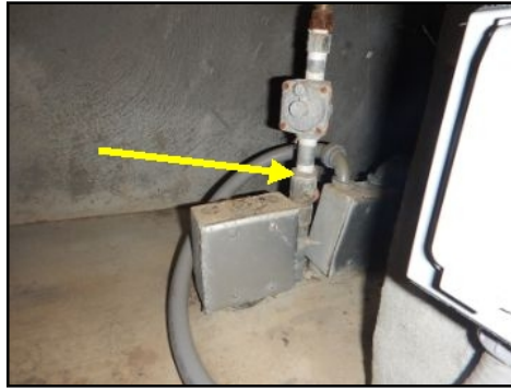
FYI - Gas shut-off valve under outdoor grill
