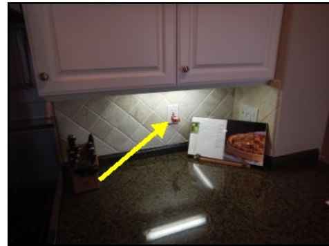
Faulty GFCI receptacle on kitchen countertop
