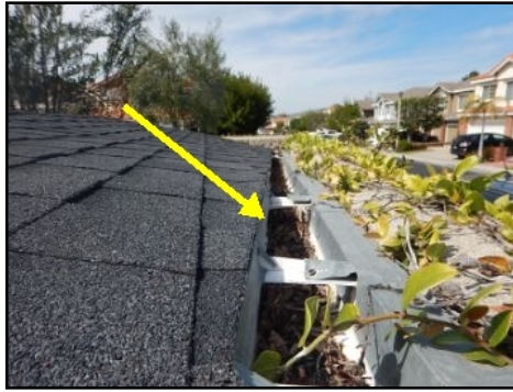
Gutter on shed needs cleaning
