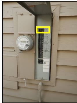
Improper 50 amp fuse for A/C
