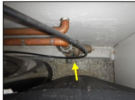
FYI - House Water Shut-off Valve
