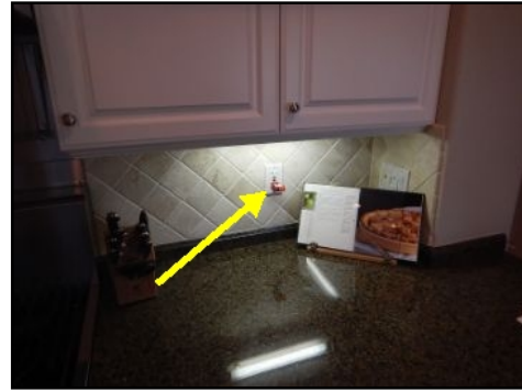
Faulty GFCI receptacle on kitchen countertop
