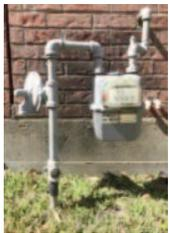
A Brightwater resident discovered that his outside gas piping was leaking. A gas leak smells like rotten eggs or sulfur. He called CenterPoint Energy, and they replaced the valve and meter. The next day, he smelled gas outside a neighbor's home, and CenterPoint also fixed that problem. Since our homes are reaching the quarter-century mark, it's a good idea to do an odor check near your outside meter.
