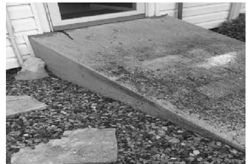
Original cement ramp
