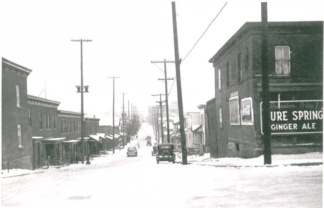
Gladstone and Rochester looking west
