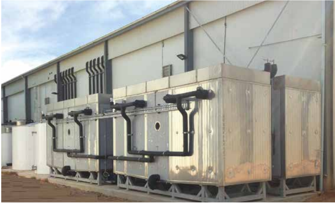
Tanks that house the specialised salt-based PCM used commercially for the first time.
