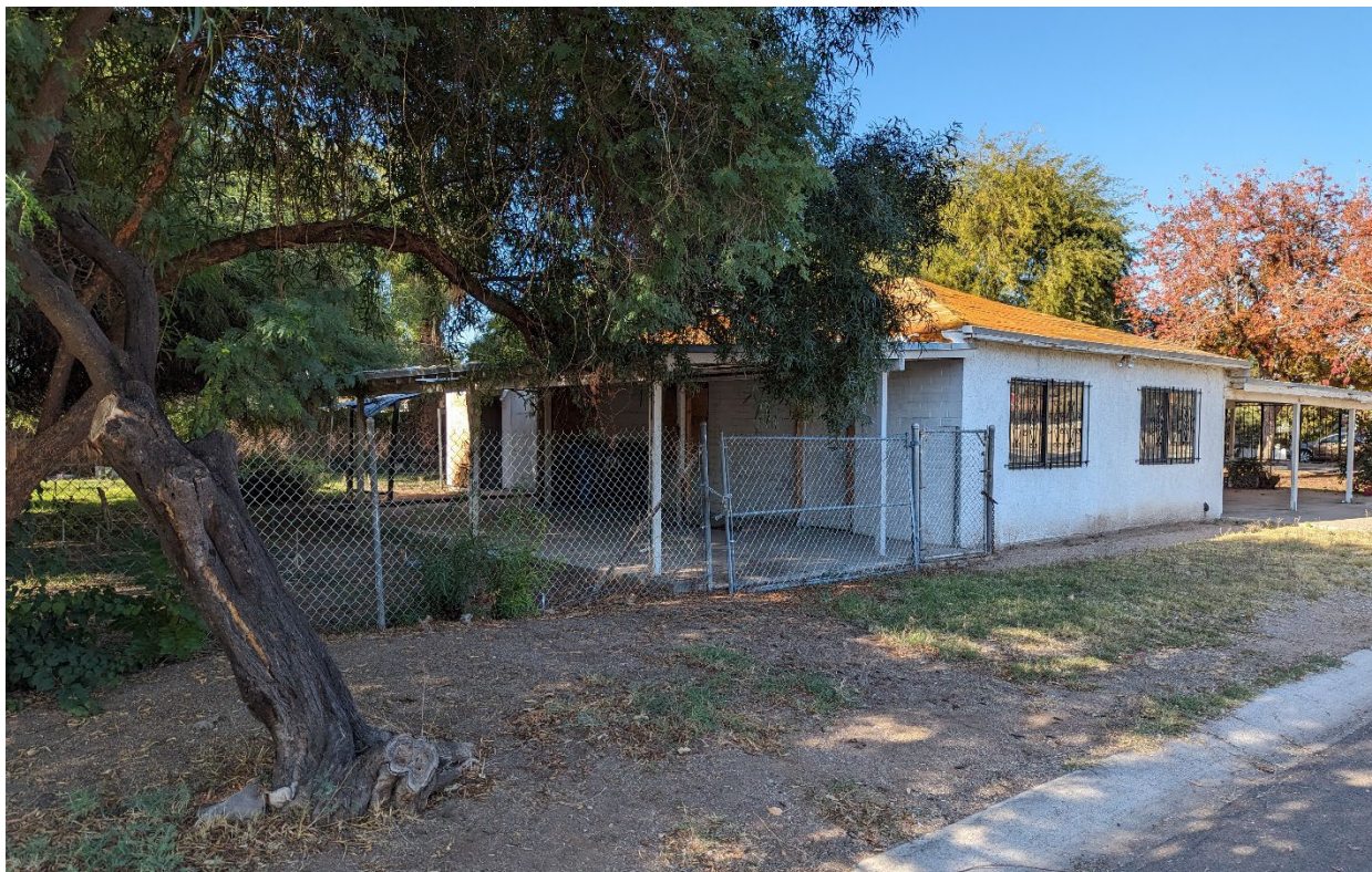
View looking northwest – approximate location of rear additions
