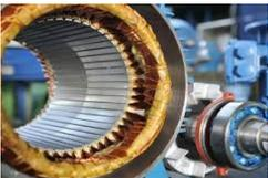
Simply put, rewinding a motor means replacing and recreating the coils of copper wire wrapped around the stator or armature. Plus, seals and bearings are replaced. It's a precise process, but can be a cost effective way to rebuild an expensive or hard to find motor. Something to consider for motors above 50 HP.
